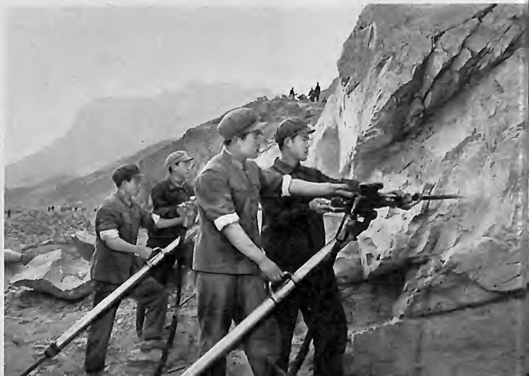
Digging a tunnel.
